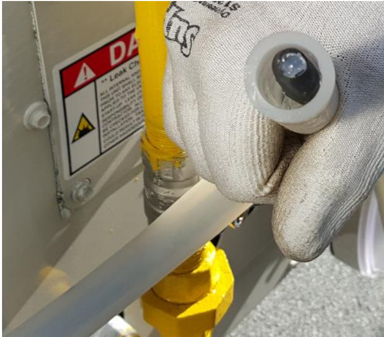
Figure 26 - Example of a heat tracing line in the condensate drain line
