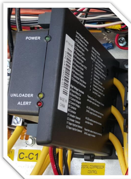
Figure 12 - Copeland digital scroll compressor controller, side and back view
