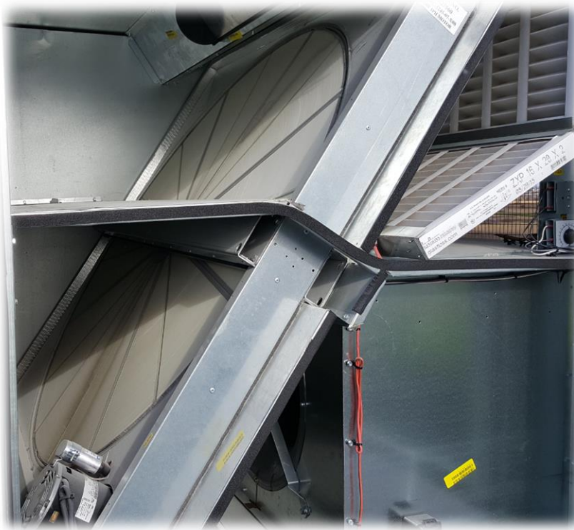
Figure 4 - Heatwheel media, motor, econ bypass damper, and fresh air filters shown
